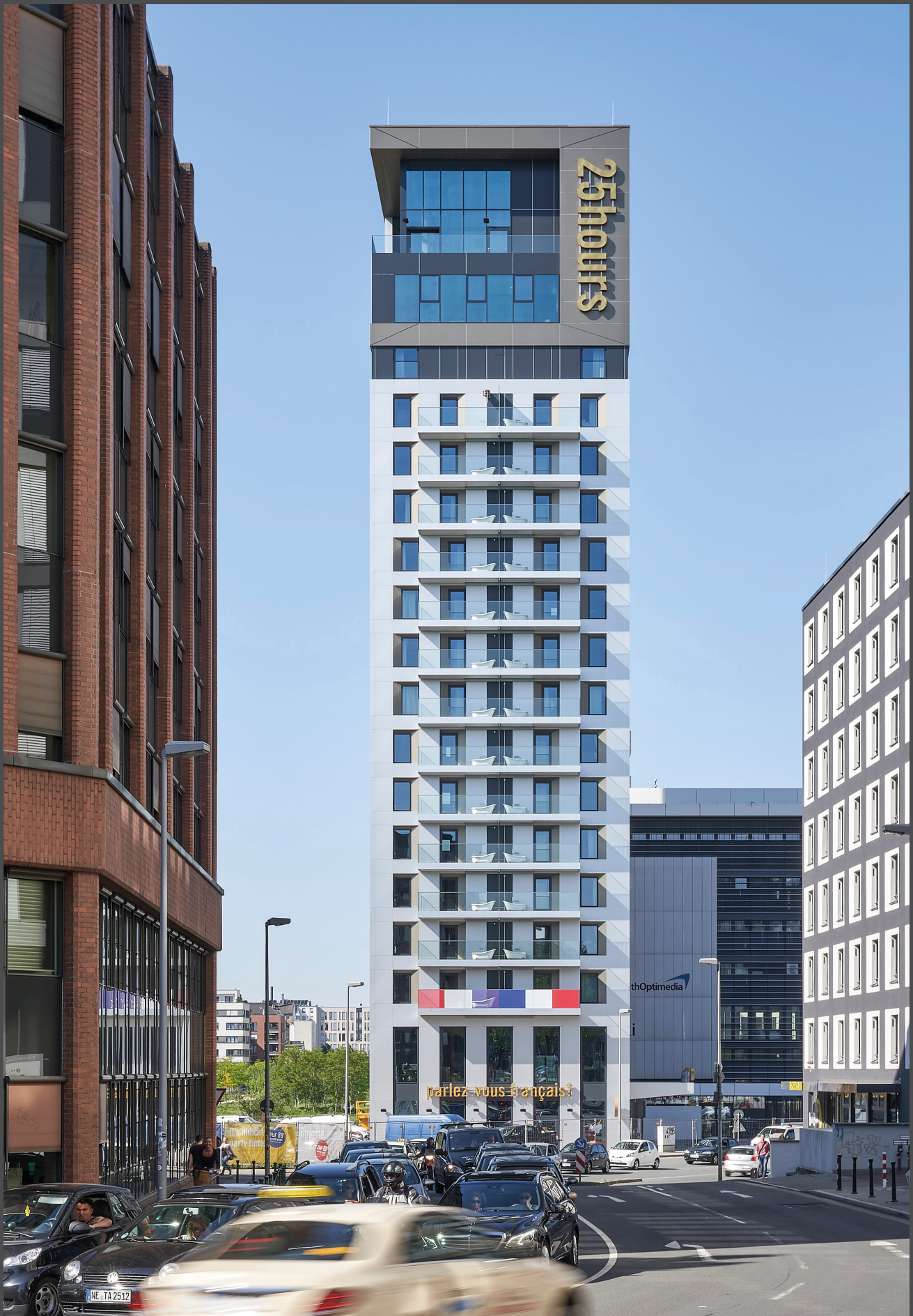
25hours Hotel Dusseldorf, Germany | Architect: HPP Architekten GmbH, Dusseldorf | Fabricator & Installer: Henke AG, Hagen | Material: ALUCOBOND® A2 anodized look C32 + C0/EV1 | © Andreas Horsky
