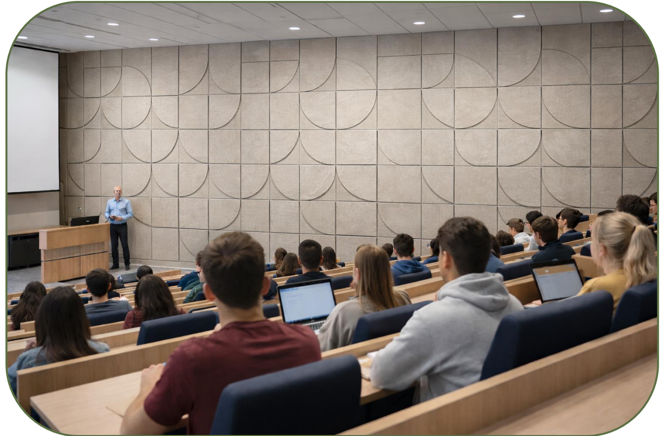
Lecture hall | Individual tiles, contour-cut elements bonded in a double-layer construction
