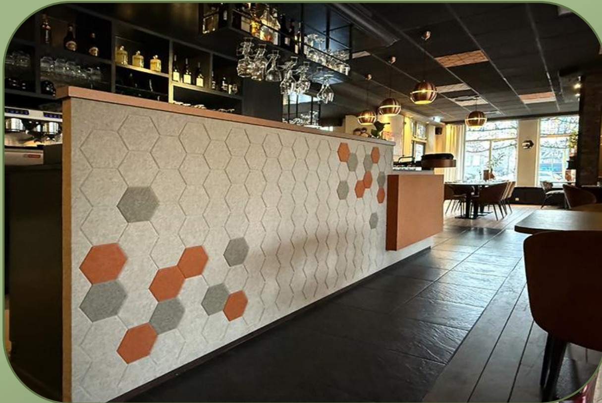
Restaurant | Panels with V-cut technique and contrasting colour inlays Design & installation by JA! Reclame & Styling
