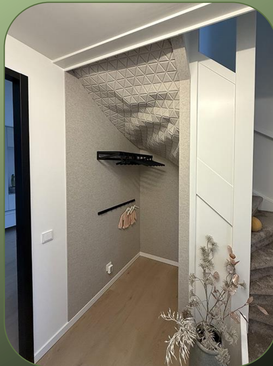
Hallway | The V-cuts allowed the felt to be shaped more easily to the stair treads.
