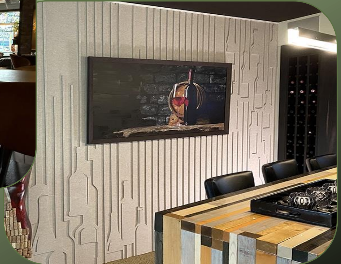
Double-layer felt, bonded together; contour-cut top layer. Design & installation by JA! Reclame & Styling
