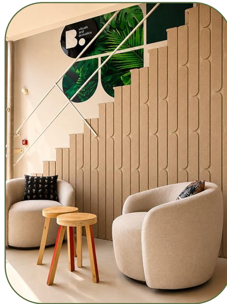
AcoFelt shapes, contour-cut and glued directly to the wall. Design & installation by Braat Visual Creations
